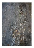
Nearby you will see a beautifully constructed cobblestone roadside water channel. This is a very attractive example of fine textured and meticulous, creative stone workmanship. It served to carry away rainwater, which prevented damage or rutting to the main avenue. A gang of workmen using knives, kept the watercourse clean during the working period of the estate.
